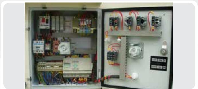
Electric panel with overload protection elements and integrated controls
